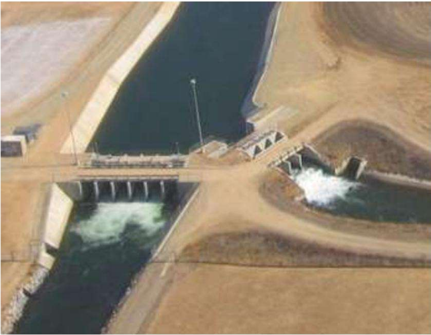
Fig1: DIVERSION HEADWORK
