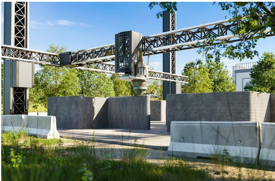
Gantry 3D printer in construction
