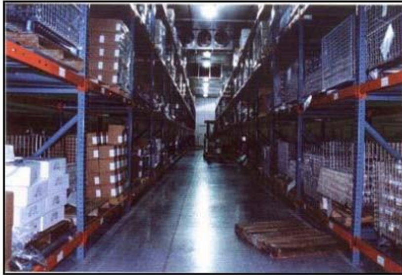
Fig.3.3. Photograph of a typical cold storage
