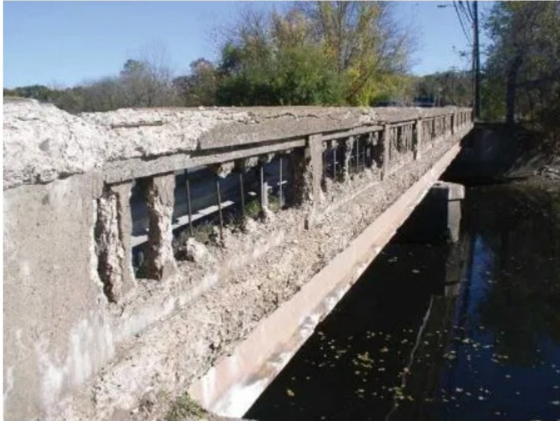
Fig 4: Freezing and Thawing Effect on Concrete
