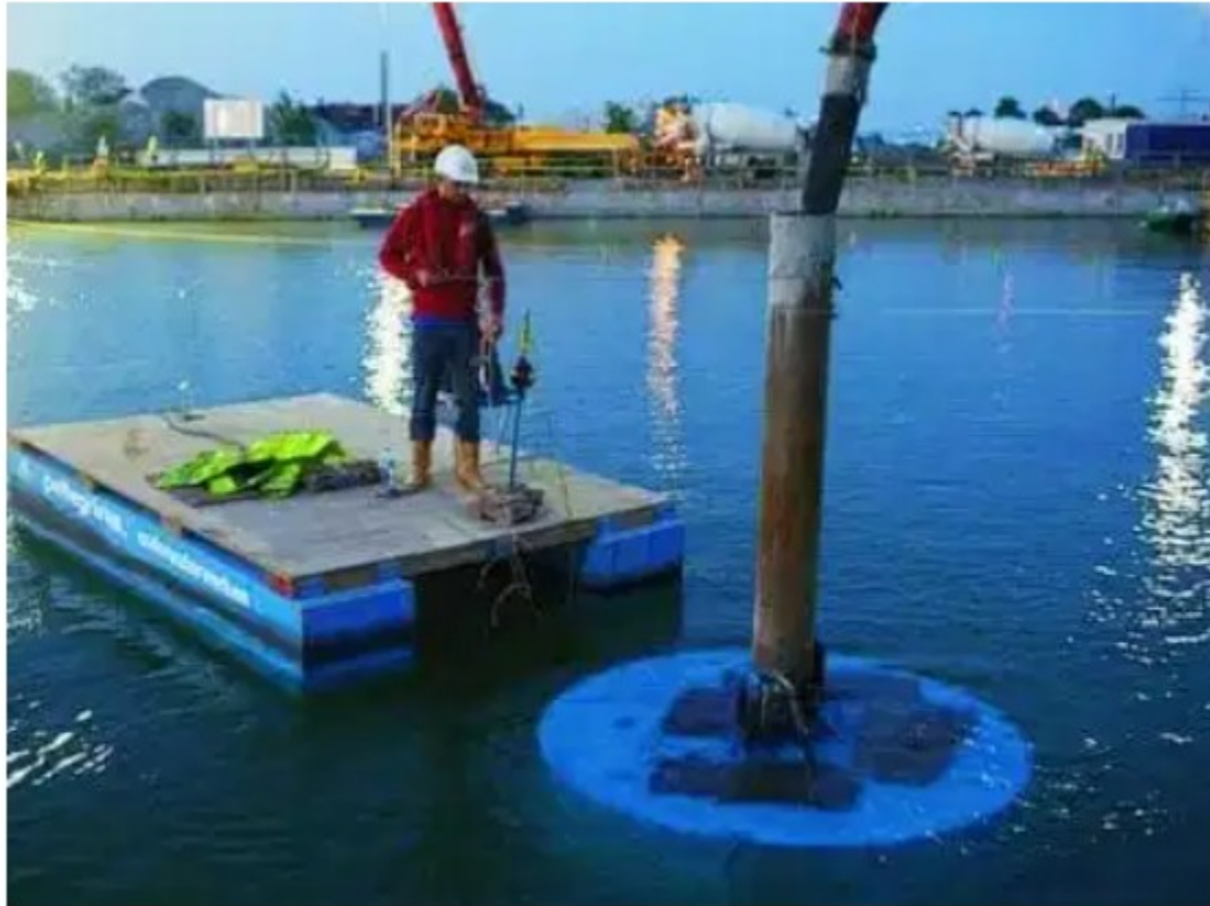
Fig 9: Underwater Concreting
