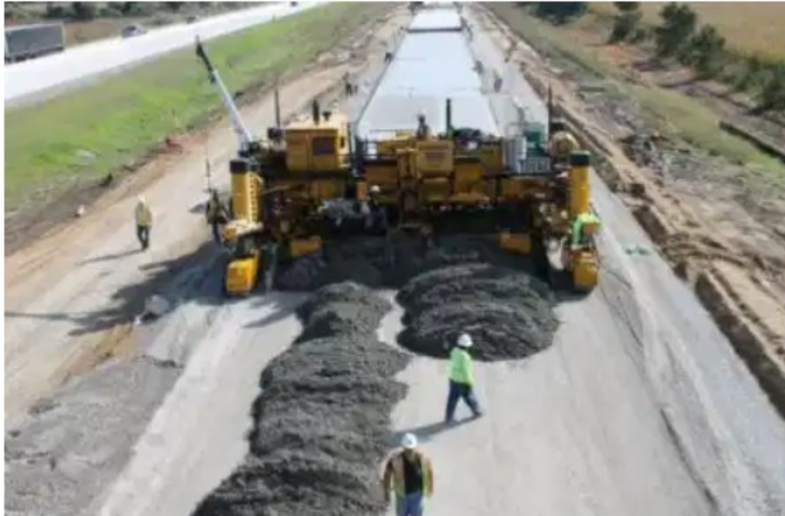
Fig 12: Concrete Pavement Overlay
