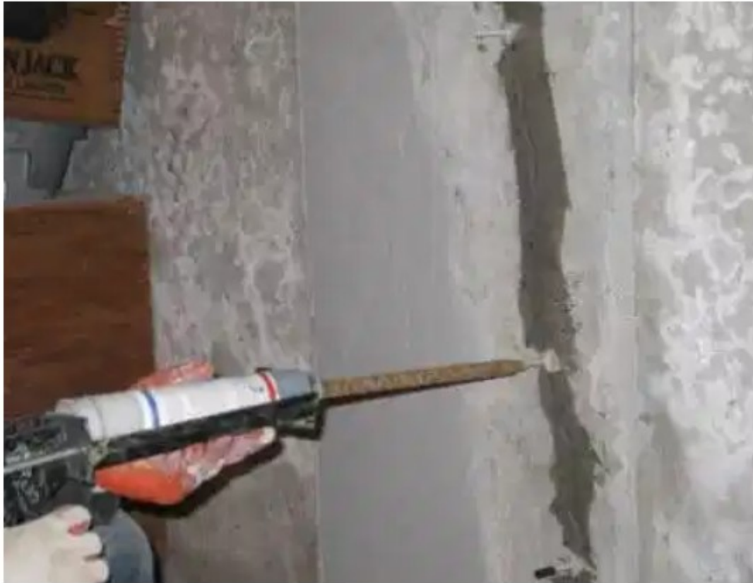
Fig 10: Grouting
