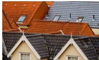
Maximizing Your Space with a Sloping Roof
