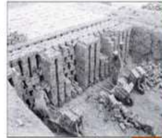
A Bull's trench kiln with a fixed chimney
