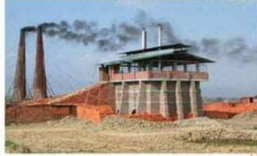
Vertical Shaft Brick Kiln
