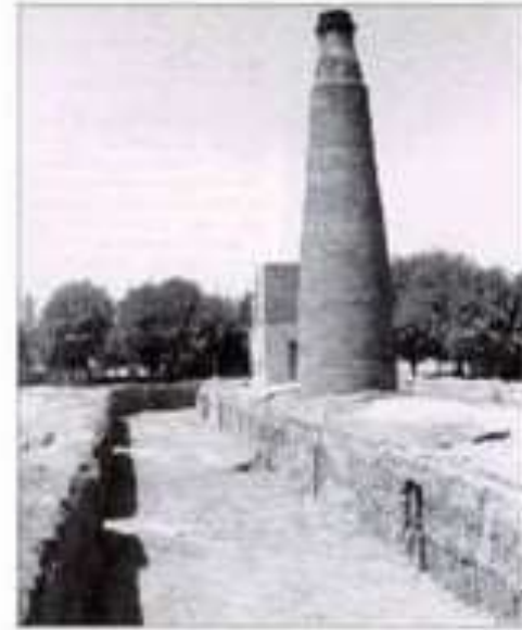
A Bull's trench kiln with a fixed chimney
