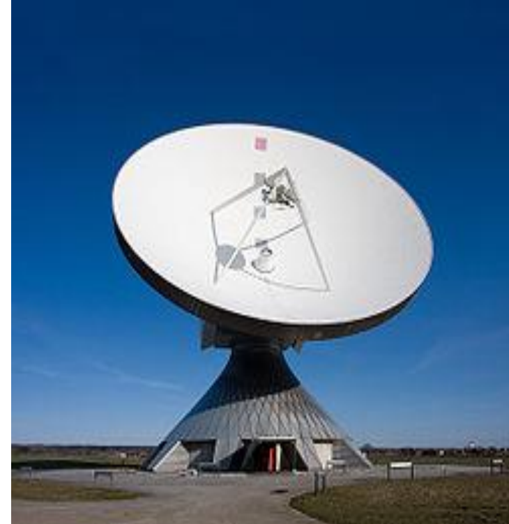
Figure : Parabolic Antenna
