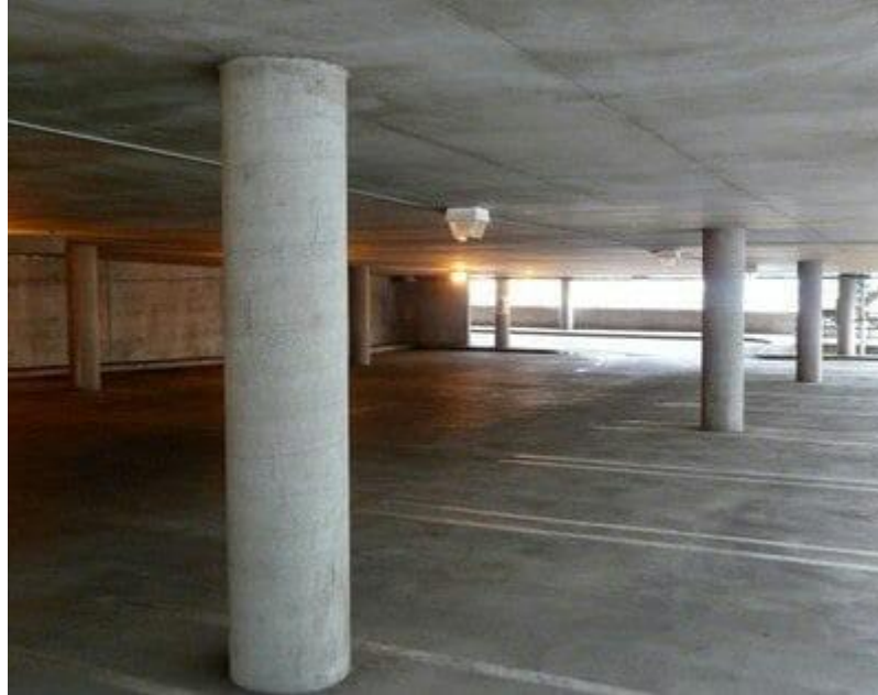
Flat plate floor system
