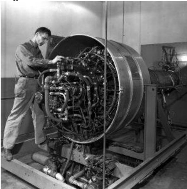
A mechanic works on a General Electric I-40 engine installed in Cell No. 3 of the JPSL (1946).
