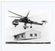
A Sikorsky S-64 Skycrane lifting a prefab house
