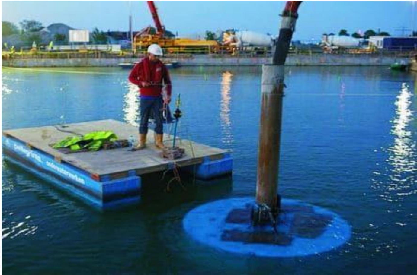
Fig 9: Underwater Concreting
