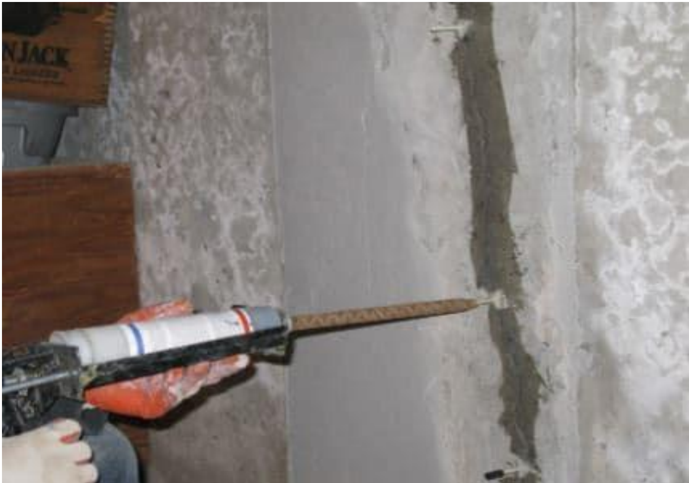
Fig 10: Grouting
