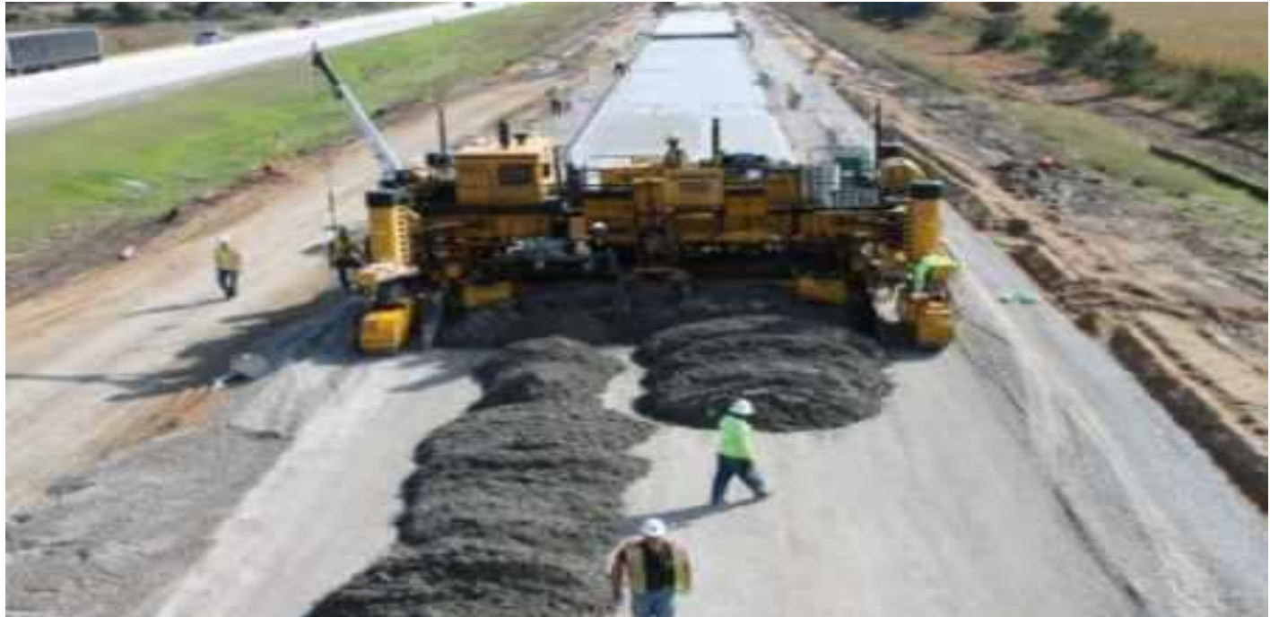
Fig 12: Concrete Pavement Overlay
