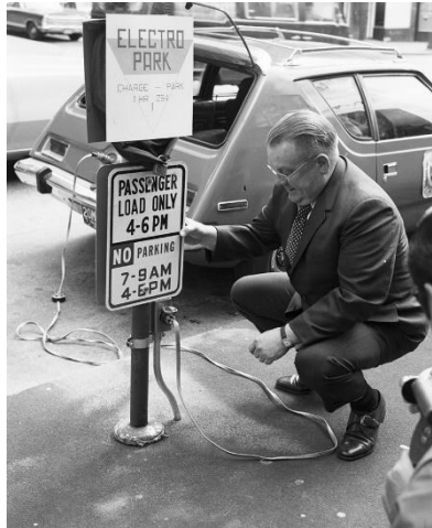
Charging station with NEMA connector for electric AMC Gremlin used by Seattle City Light in 1973
