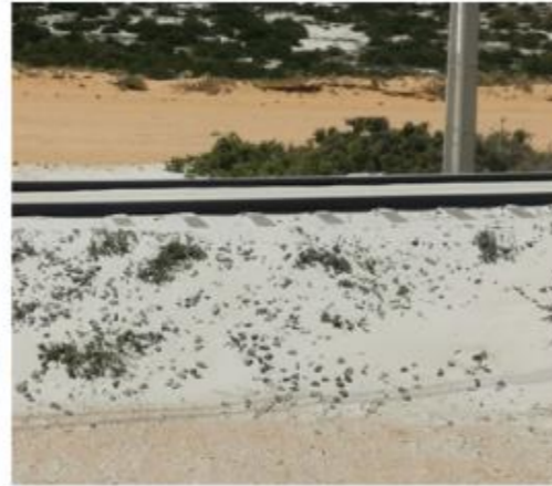
(B) Sand Sedimentation on Track
