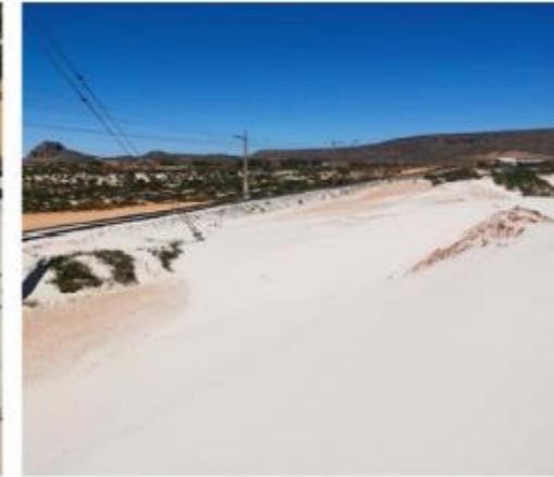
(C) Sand Build-Up on Heavy Haul Line
