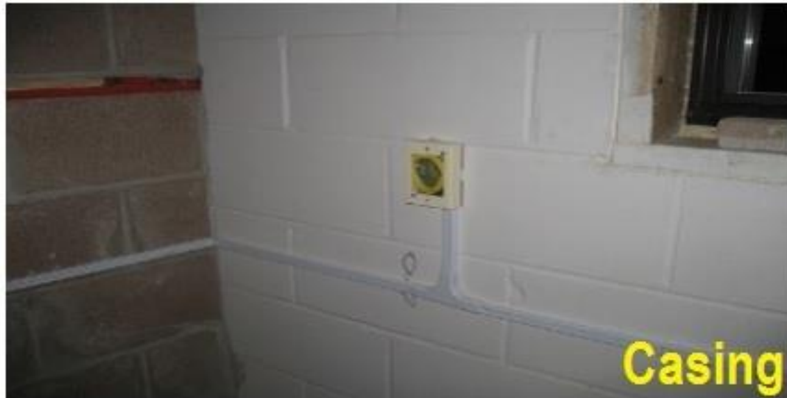
Casing and Capping Electrical Wiring
