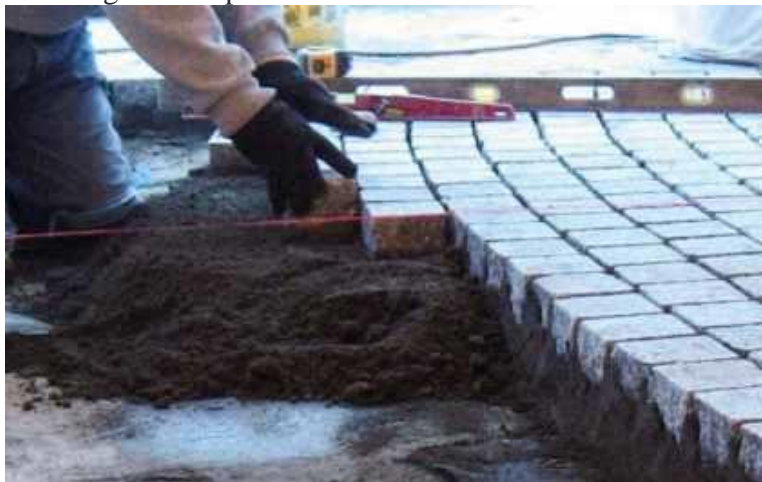
Fig. 4: Setting Bed for Installation of Bricks
