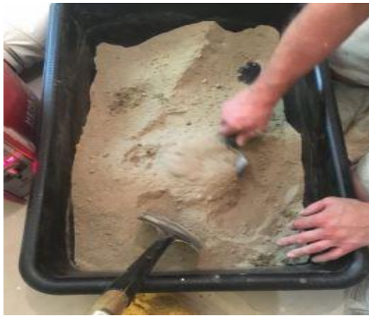
Fig. 2: Dry Pack Mortar Before Adding Water
