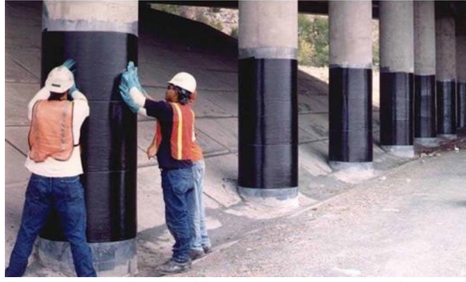
Figure 4- Hoop tension in CFRP- strengthened circular column
