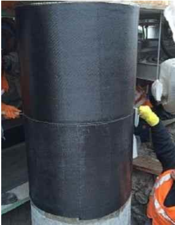
Fig. 3: Wrapping RC Columns with CFRP
